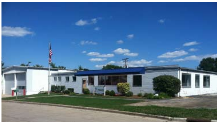
Trinity's Waukesha, Wisconsin facility (picture file attached)
